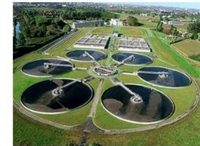
Waste Water Treatment
